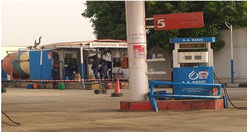
Plate 2: Add-on Skid Modular at A.A. Rano Filling Station at 3 rd Gate along Gwarzo Road
